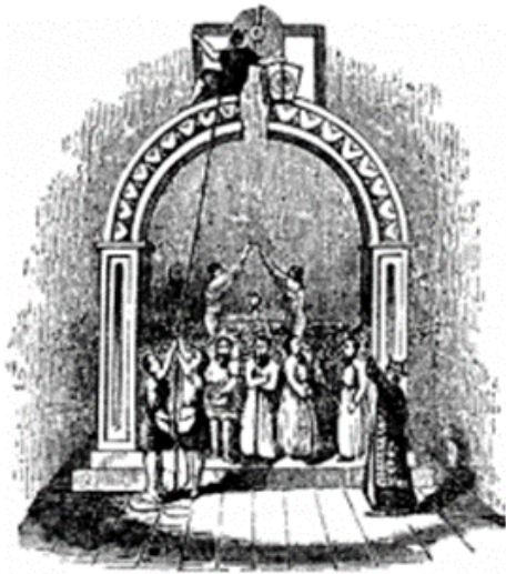
Figure 52 - The Keystone set in place
