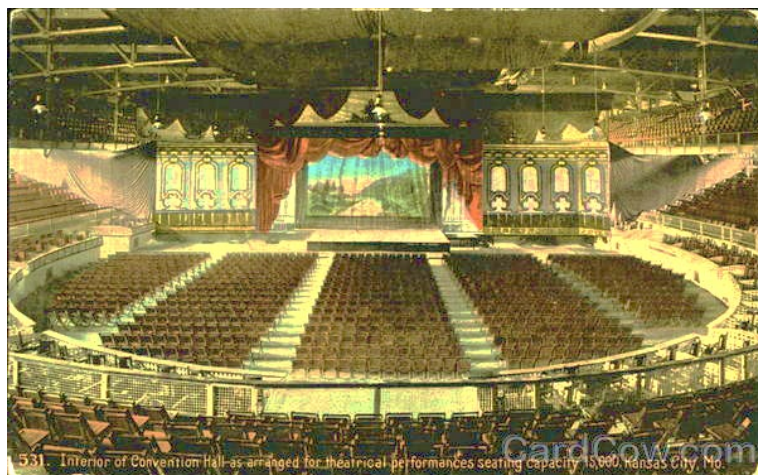
Figure 48 - Interior of Old Convention Hall, Kansas City
